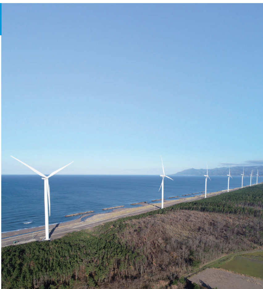
某風力発電所 (3,200kW×7基) Wind power station (3,200 kW × 7 units)
