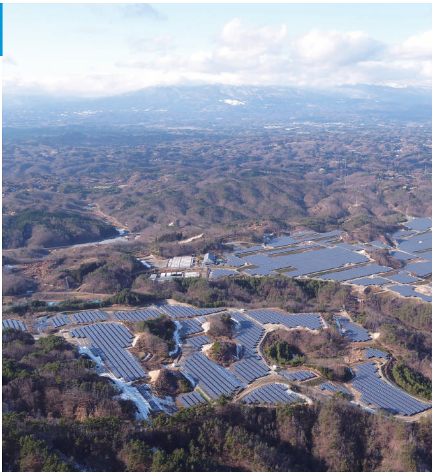
某太陽光発電所 (29,508kW) Photovoltaic power station (29,508 kW)
