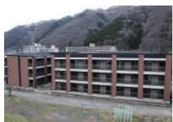
釜石市上中島町復興住宅 (岩手県釜石市) Kamaishi City Kaminakashima-cho restoration housing (Kamaishi City, Iwate Prefecture)
