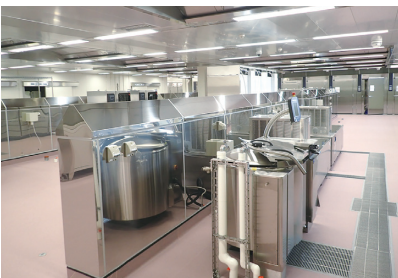
Kitchen equipped with a ceiling ventilation system (top of the photo)
