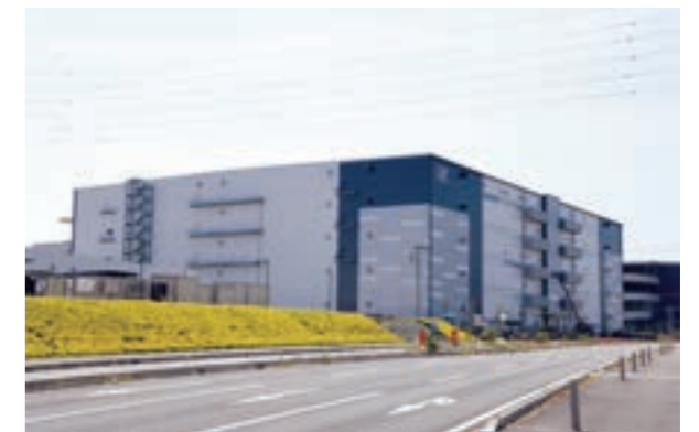
LF Tsukuba (large-scale logistics center) (Ibaraki Prefecture)
