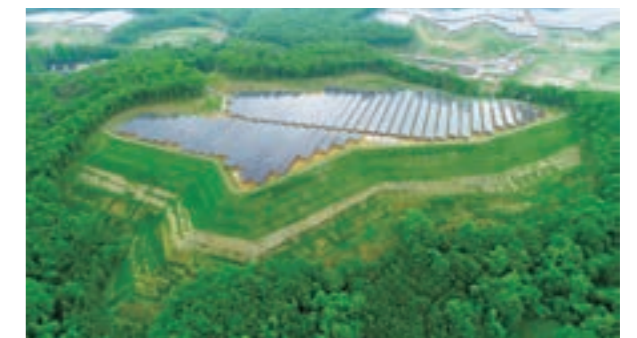
Miyagi Kawasaki Solar Power Plant (Miyagi Prefecture)
