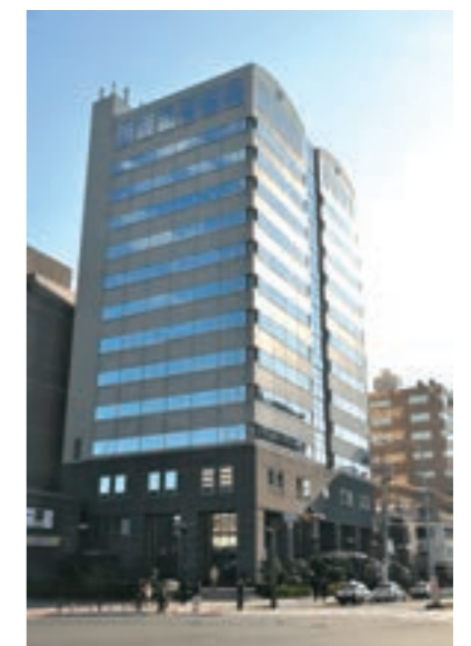
Head Office Building Sendai City, Miyagi Prefecture
