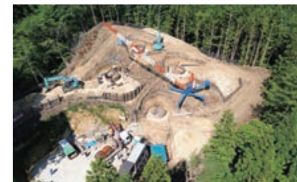
Miyagi Marumori Main Line steel tower foundation work (Miyagi Prefecture)
