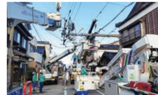
2024 Noto Peninsula Earthquake restoration work (Ishikawa Prefecture)
