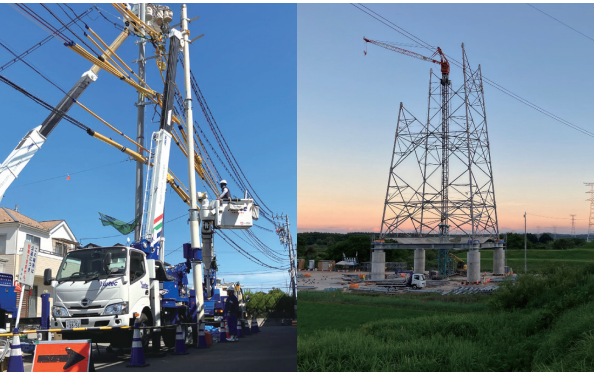
Improving utility pole replacement efficiency (Utility pole base location reconstruction vehicle) (Miyagi Prefecture) Construction of new steel towers for the Dewa Main Line (Akita Prefecture)
