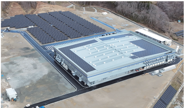
Construction of a solar power generation facility at Himeji Rika Corporation's Tamura Plant (Fukushima Prefecture)
