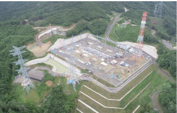
Construction of the new Miyagi Marumori switching station (Miyagi Prefecture)
