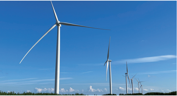
Construction of Mutsu-Ogawara Wind Farm (Aomori Prefecture)>
